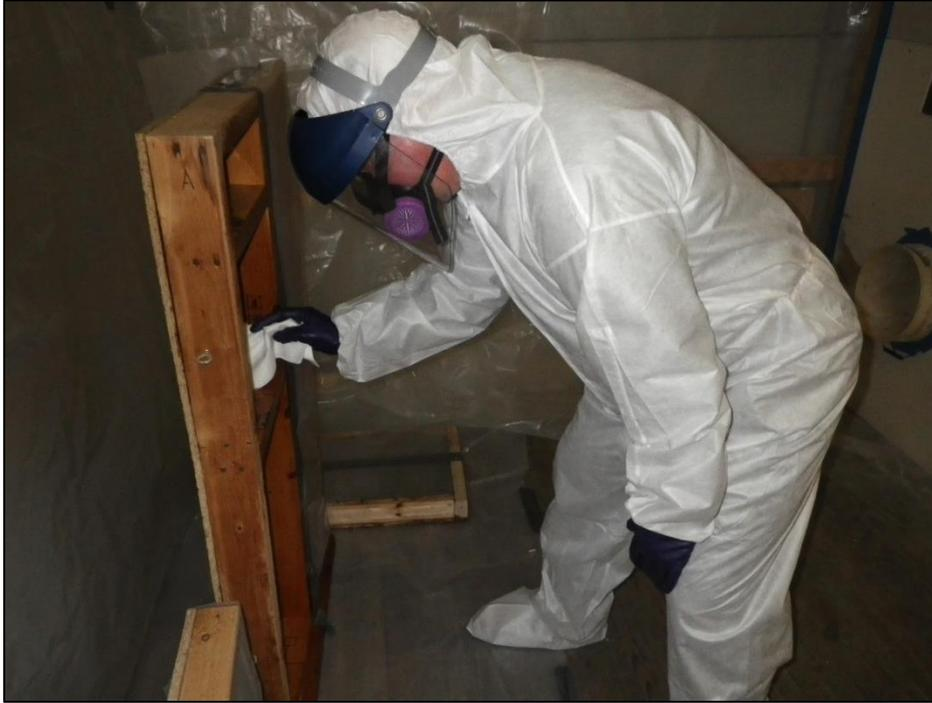
6. Following application of Atomic Degreaser, the surfaces were cleaned with disposable towels. Then Decon 30 was sprayed on the surfaces using the FOAM-iT sprayer.
