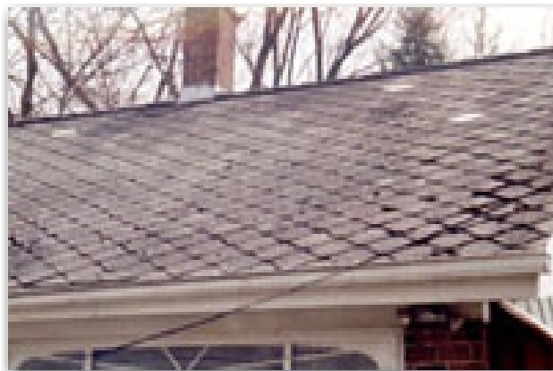
Asbestos roofing materials
