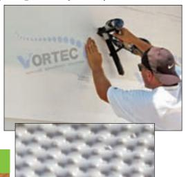
drainage of moisture in wall cavities. Vortee is a thin, flexible plastic film micro-perforated and engineered with a pattern of dimples and bumps that is installed on the exterior of a home or commercial building during construction. The engineered-surface facilitates water drainage by channeling water that gets past the siding, away from a structure's exterior wall surface, thereby reducing the chance of mold and mildew.
