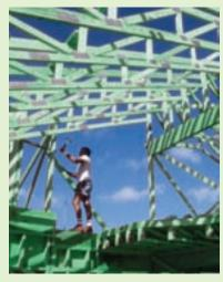
strand lumber, laminated veneer lumber and wood l-beams. The coating is readily identified by a green colorant mixed in with the active ingredients.
