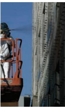
Barriseal is a water-based asphalt emulsion modified with a blend of synthetic rubbers and special additives, which cures to form a flexible, monolithic air/vapor barrier for many substrates in eavity wall construction.
