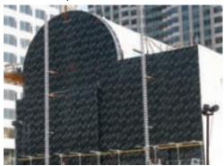
Perm-A-Barrier VP is designed for use in wall assemblies above grade and is suitable for new and remedial commercial and residential construction. It is applied by spraying it directly onto substrates. According to the company, this application method requires minimal surface preparation and eliminates the need for fastener holes that can promote air and water penetration.
