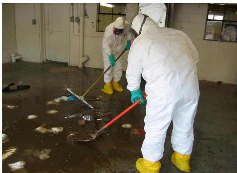
Gathering the proper tools to remove contents, muck out buildings, demolish interior surface materials, and decontaminate structural members is also important. Some tools to consider bringing to the work sites include:
